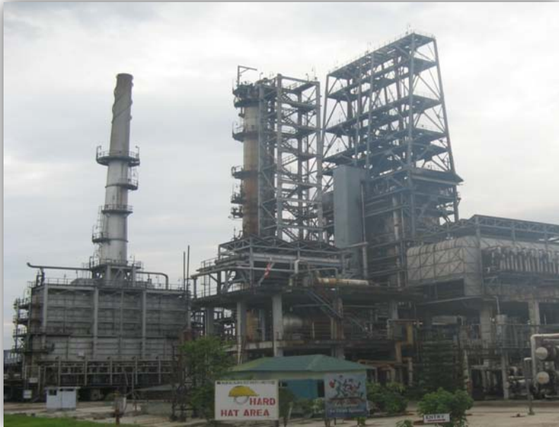
Delayed coker unit in Numaligarh Refinery
