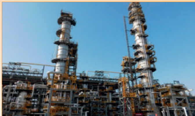
The Benzene Recovery unit (BRU)
