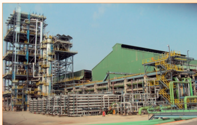
A view of the Numaligarh Refinery's Wax Plant
