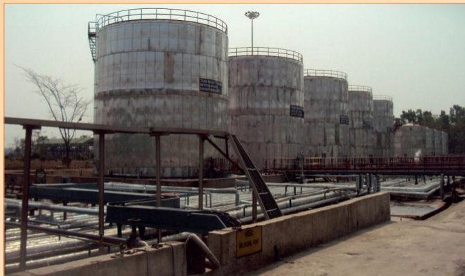
Another view of the Plant
